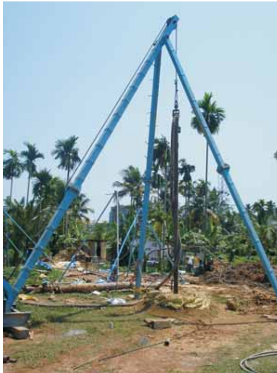
Piling Work in Progress
